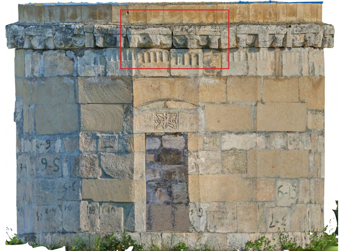
Fig. 6. Ortho-image of the mausoleum's southern facade (Iconem 2021)
