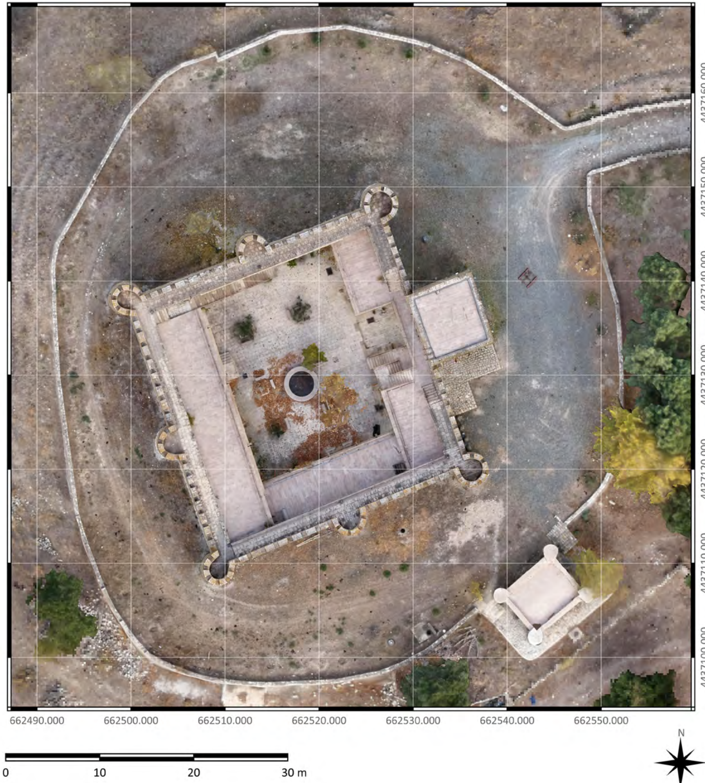
Fig. 3. Georeferenced ortho-image of Shahbulag castle extracted from the textured 3D scan (Iconem 2021)
