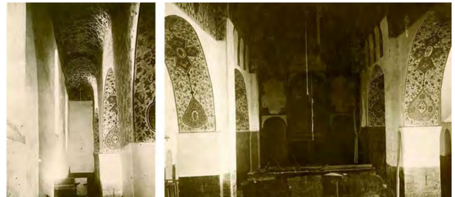
Fig. 6. Inside view of the church in 1932 (Photography of P. Grigoryan, from Avetisyan 2020, fig. 2-3)
