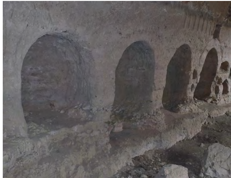
Fig. 5. The niches carved into the north-western wall (Iconem 2020)
