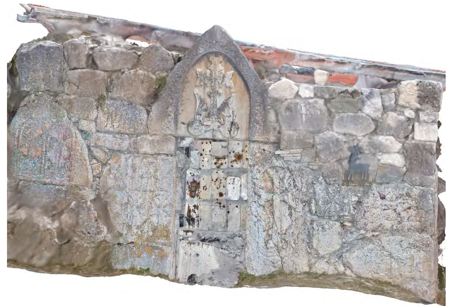
Fig. 5. Orthoimage of the western facade (Iconem 2021)
