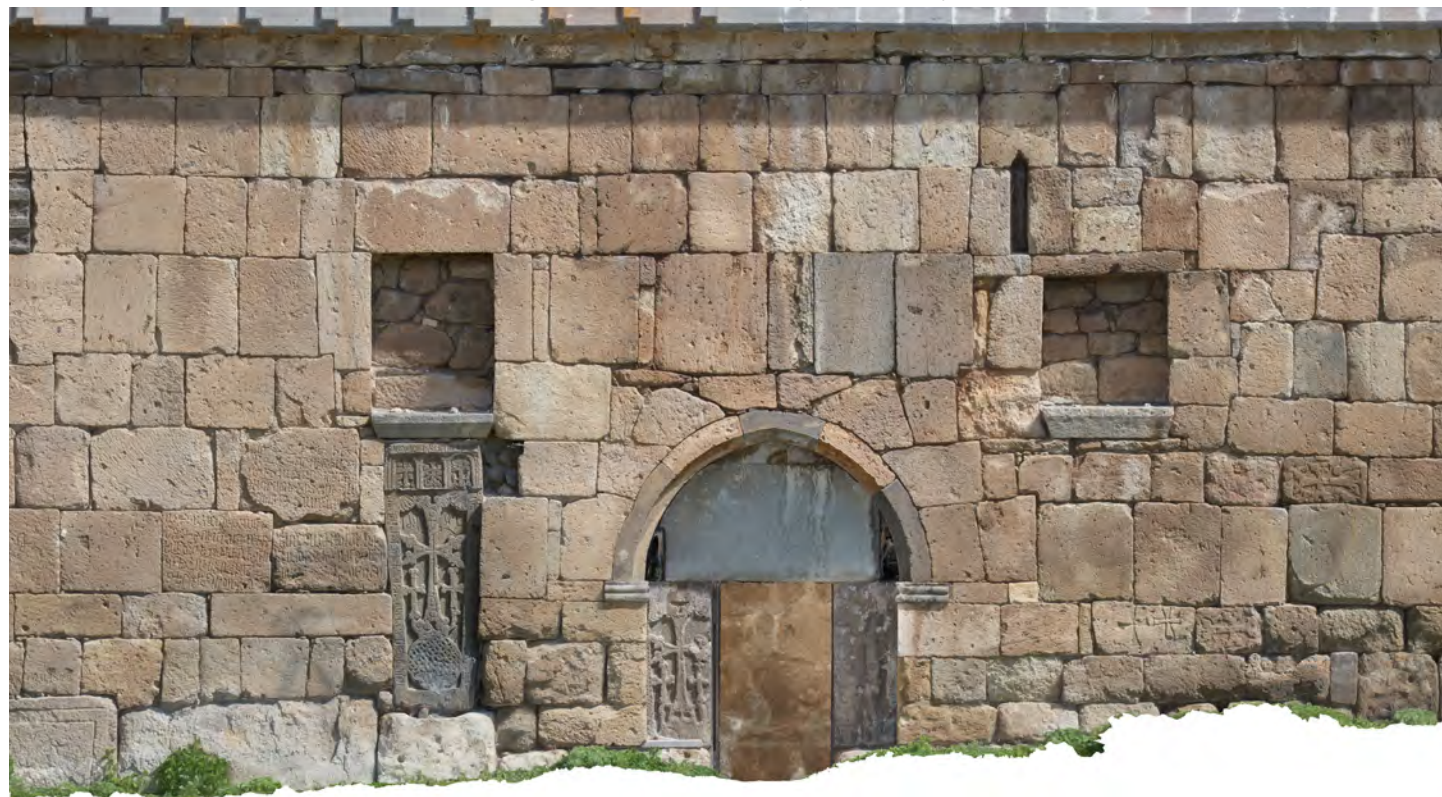
Fig. 4. Ortho-image of the Southern Façade extracted from the textured 3D scan (Iconem 2021)
