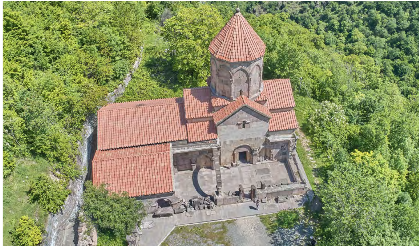
Fig. 3. Aerial view of the monastery of Vahanavank (Iconem 2021)
