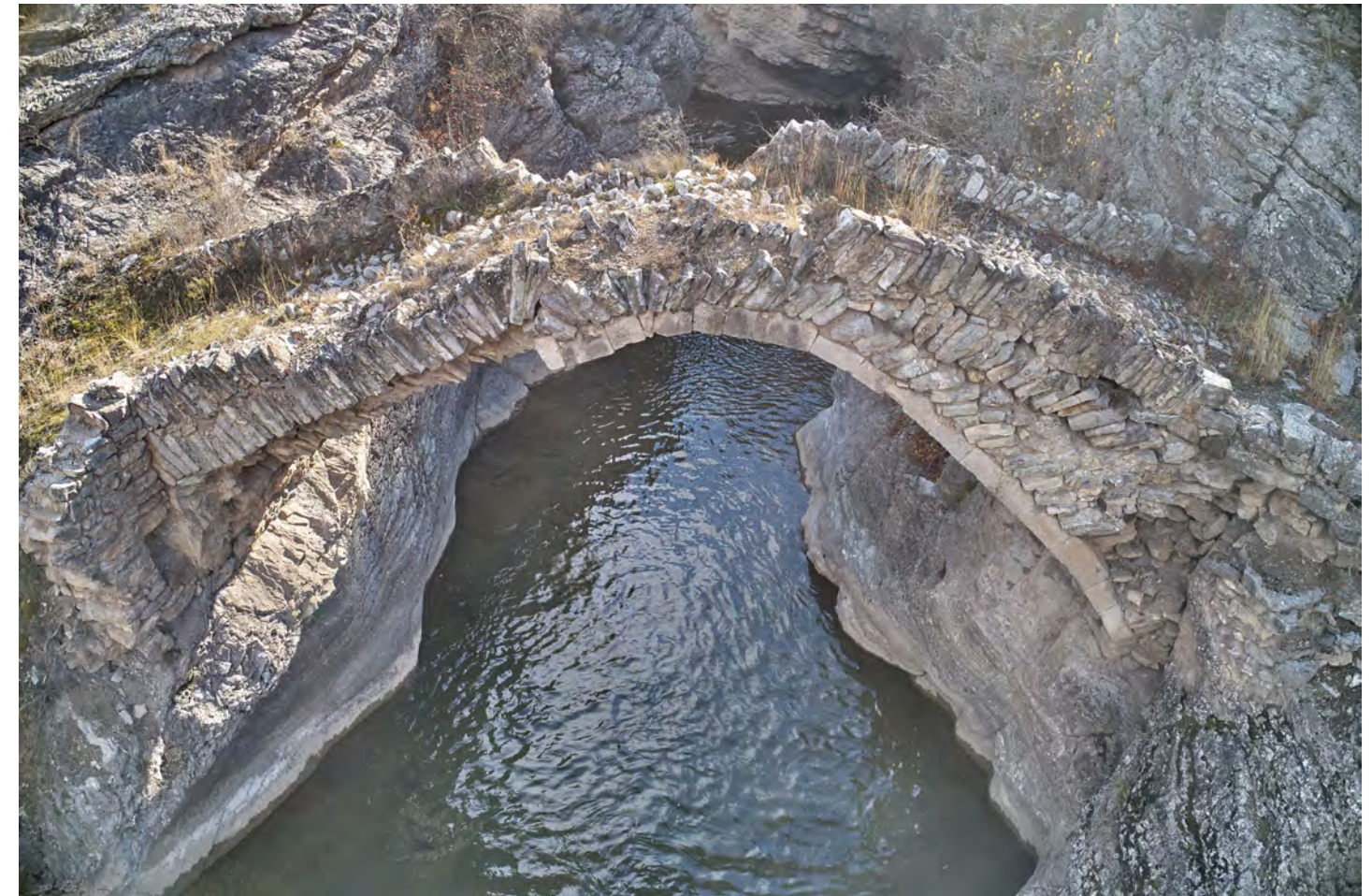
Fig. 2. Aerial view of Gandza bridge (Iconem 2020)
