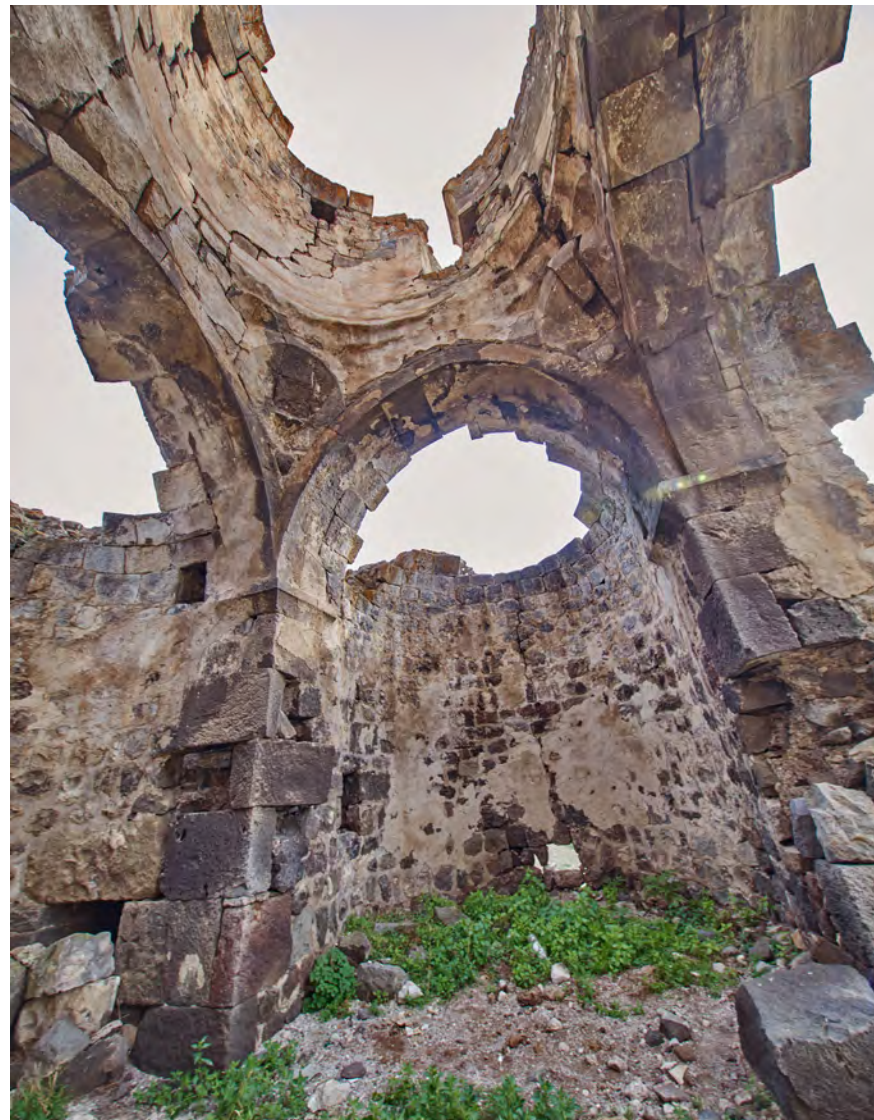
Fig. 7. The church's elevation from inside facing the eastern apse (Iconem 2020)
