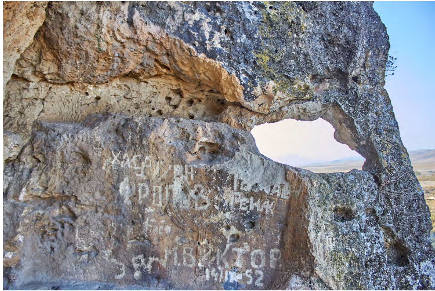
Fig. 7. View of the narthex's south-western wall (Iconem 2020)
