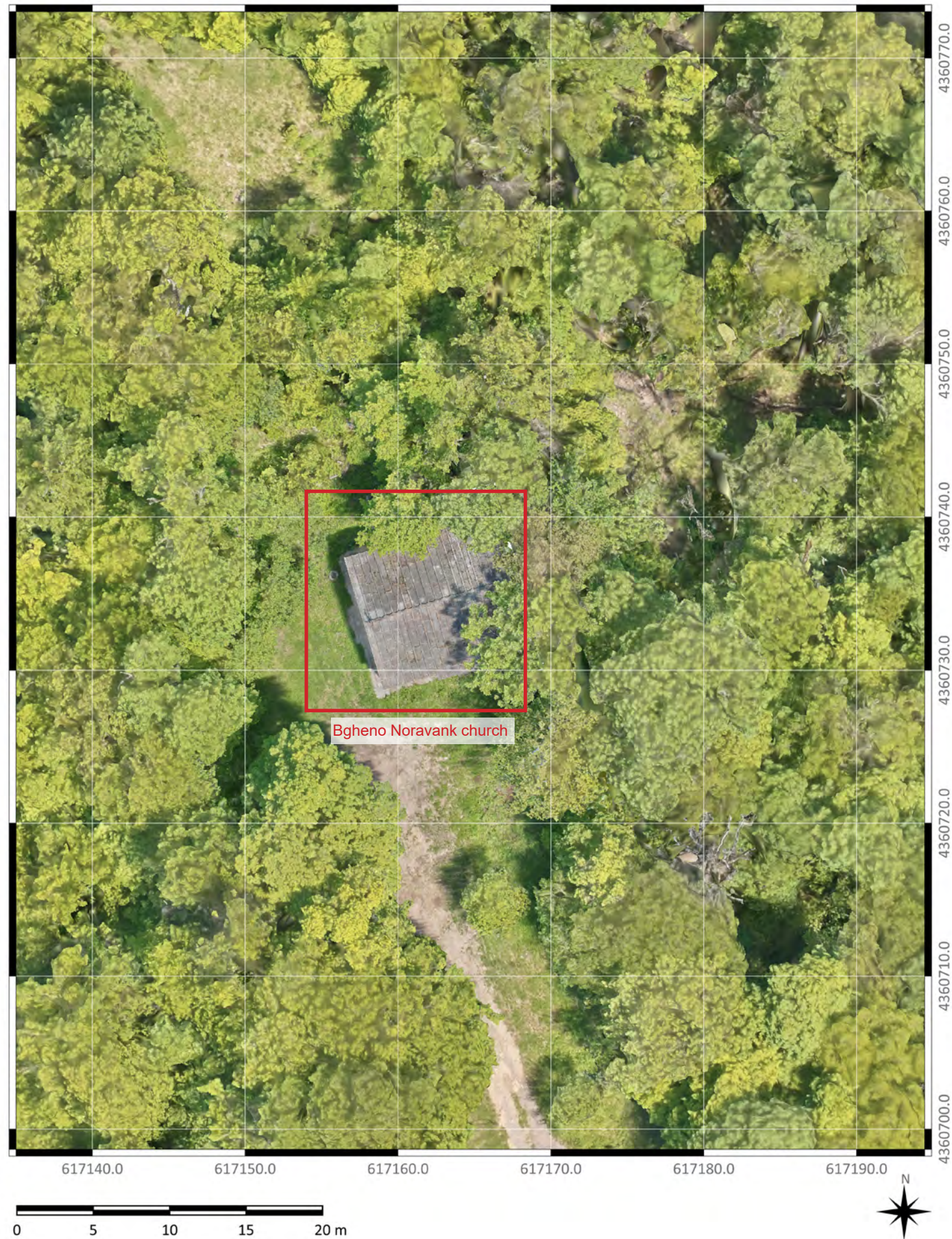
Fig. 1. Georeferenced ortho-image of the site of Bgheno Noravank monastry extracted from the textured 3D scan (Iconem 2021)
