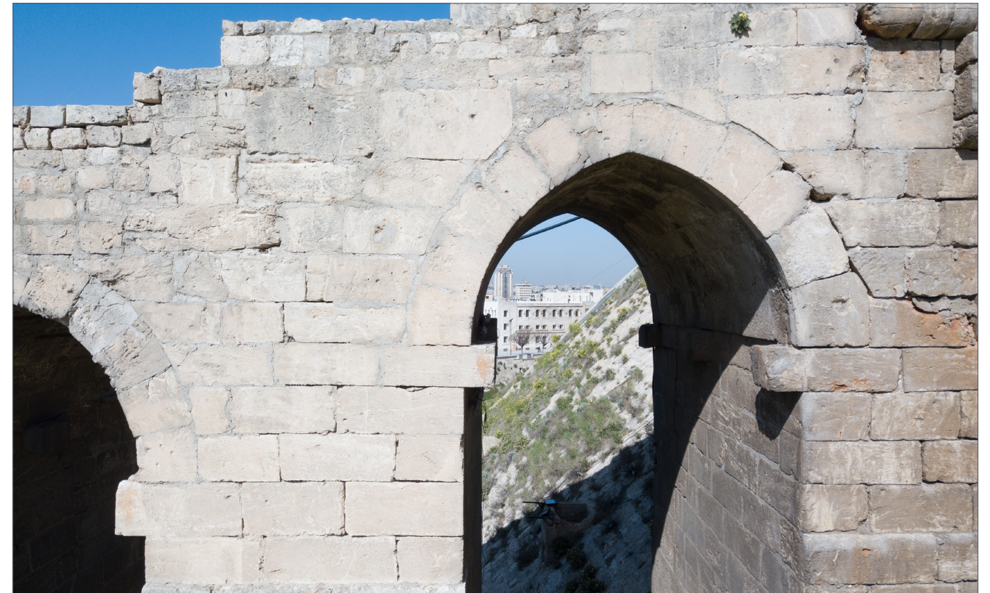
Bridge linking the outer gate (Madkhal Qal'a Halab) to the inner gate of The Citadel
