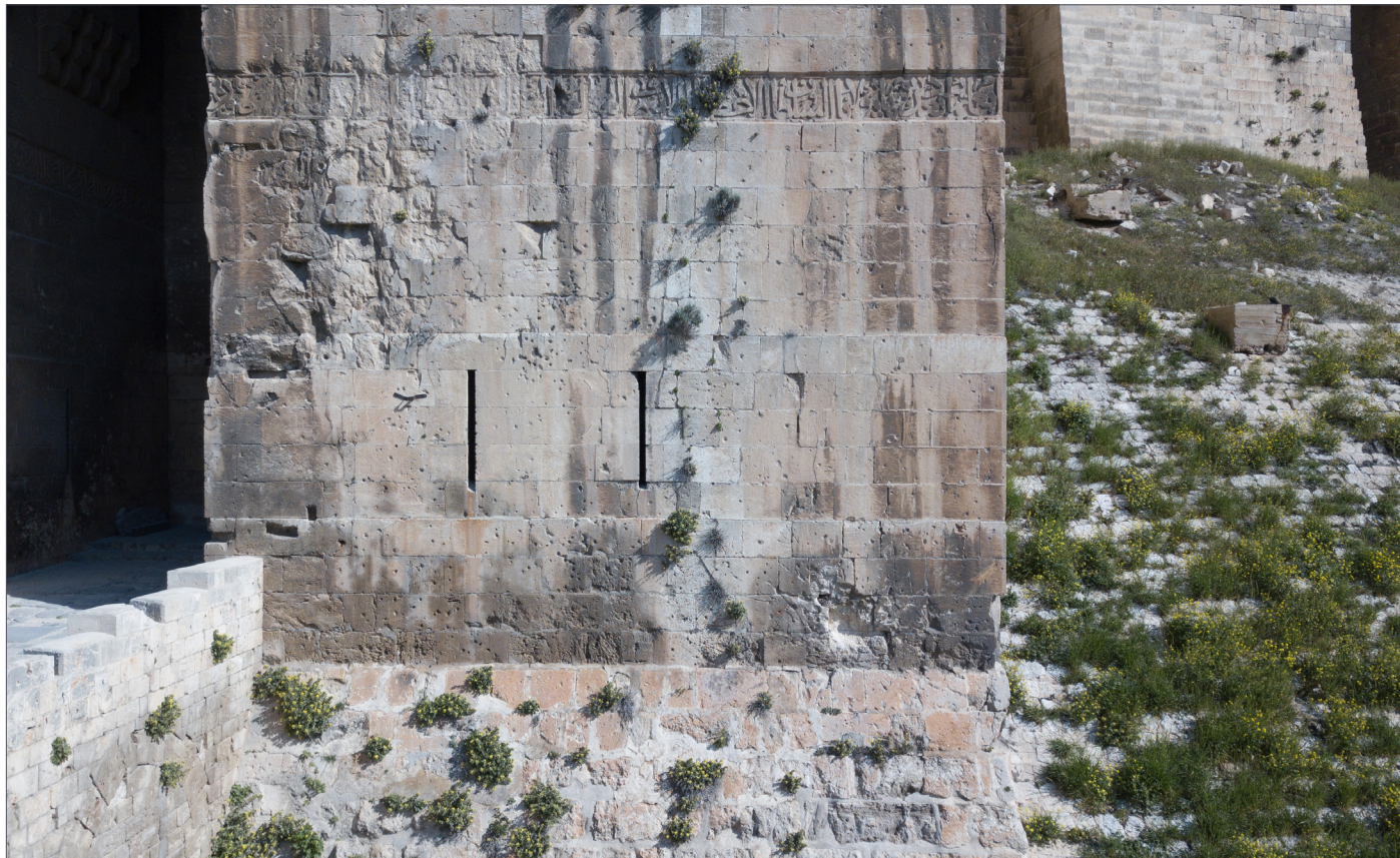
Entrance block (Madkhal Qal'a Halab) and its bridge
