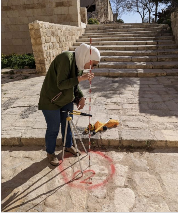
Setting up a georeferenced point
