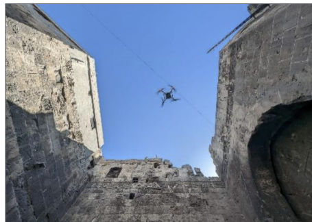
Data acquisition by drone.
